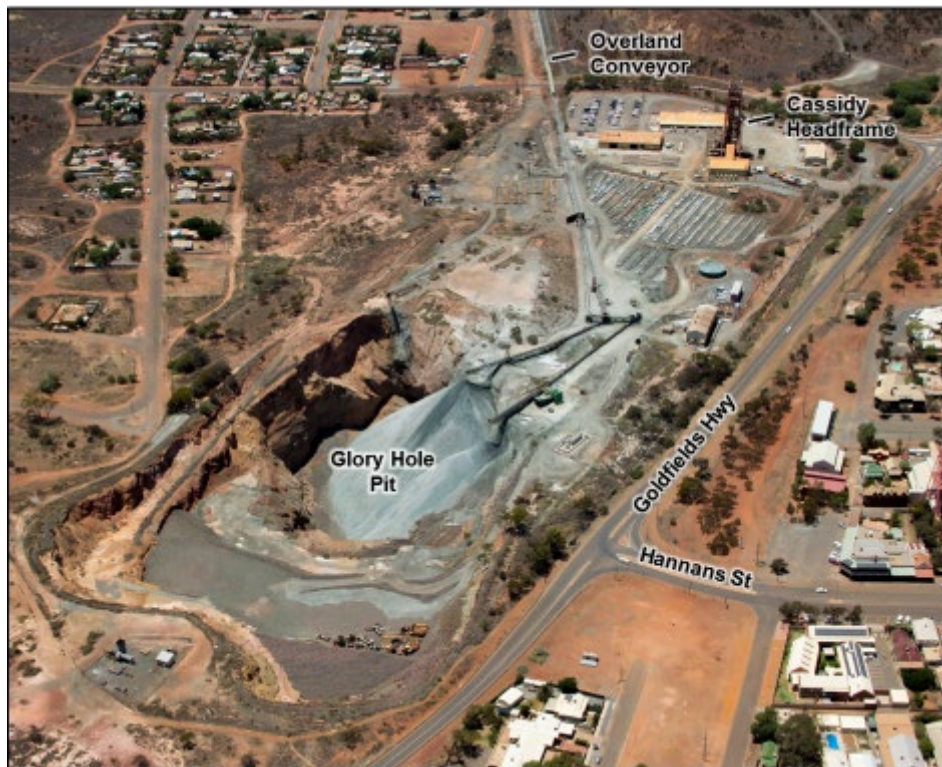
Figure 9-38: Mt Charlotte Mining Infrastructure
