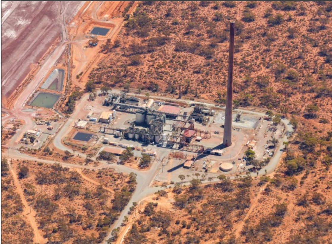
Figure 9-43: Gidji Processing Plant (2021)
