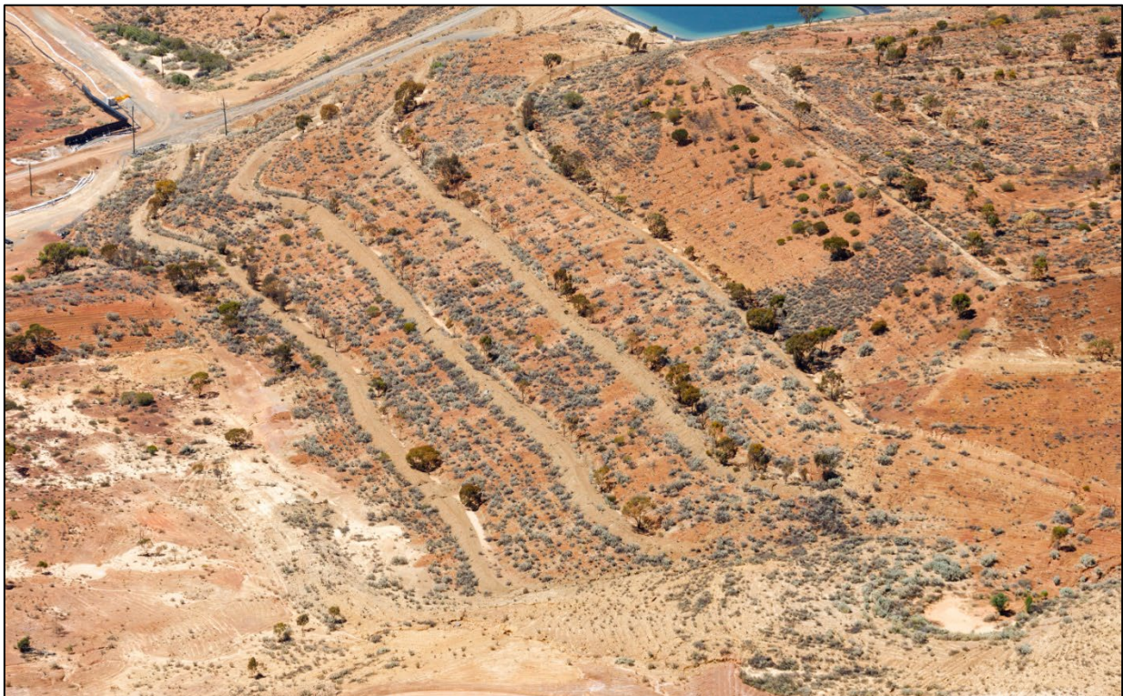
Figure 5-106: Sir John WRD Western Batter Progress of Rehabilitation
