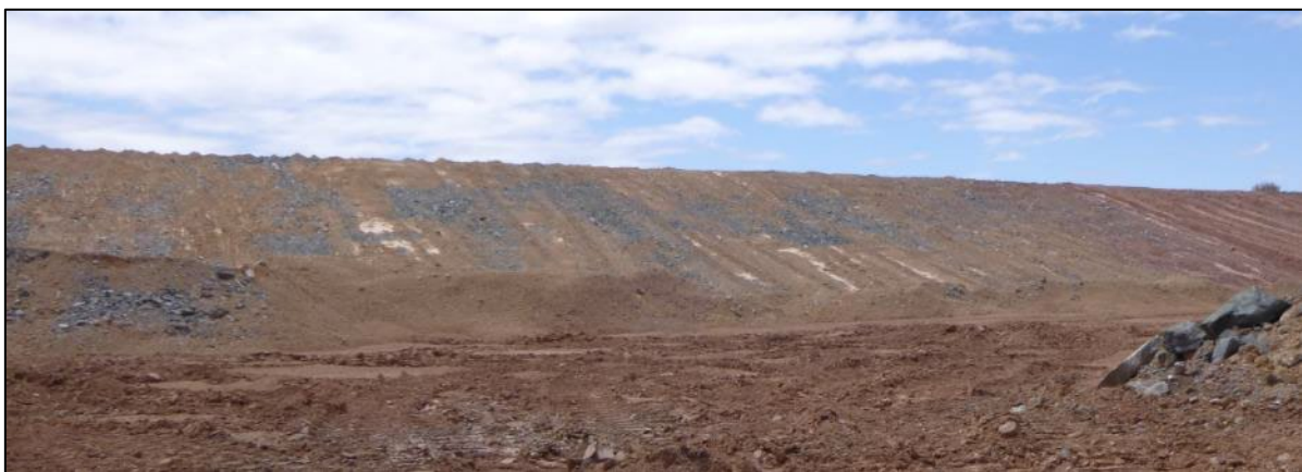
Figure 5-38: OTD Remedial Works in Progress 2017 (Oroya WRD)
