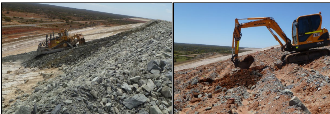
Figure 5-63: Fimiston I TSF Trial Earthworks in Progress (2016 and 2017)
