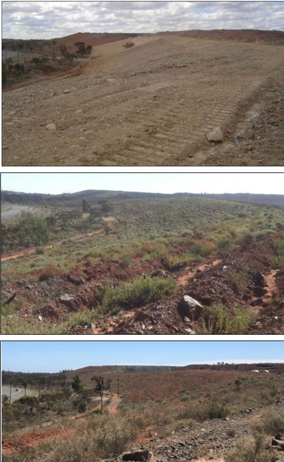
(Top: Battering 2011. Middle: 2013 Progress of rehabilitation Bottom: 2021)
