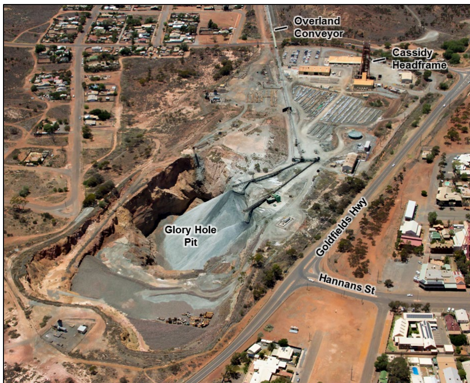
Figure 5-94: Mt Charlotte Mining Infrastructure
