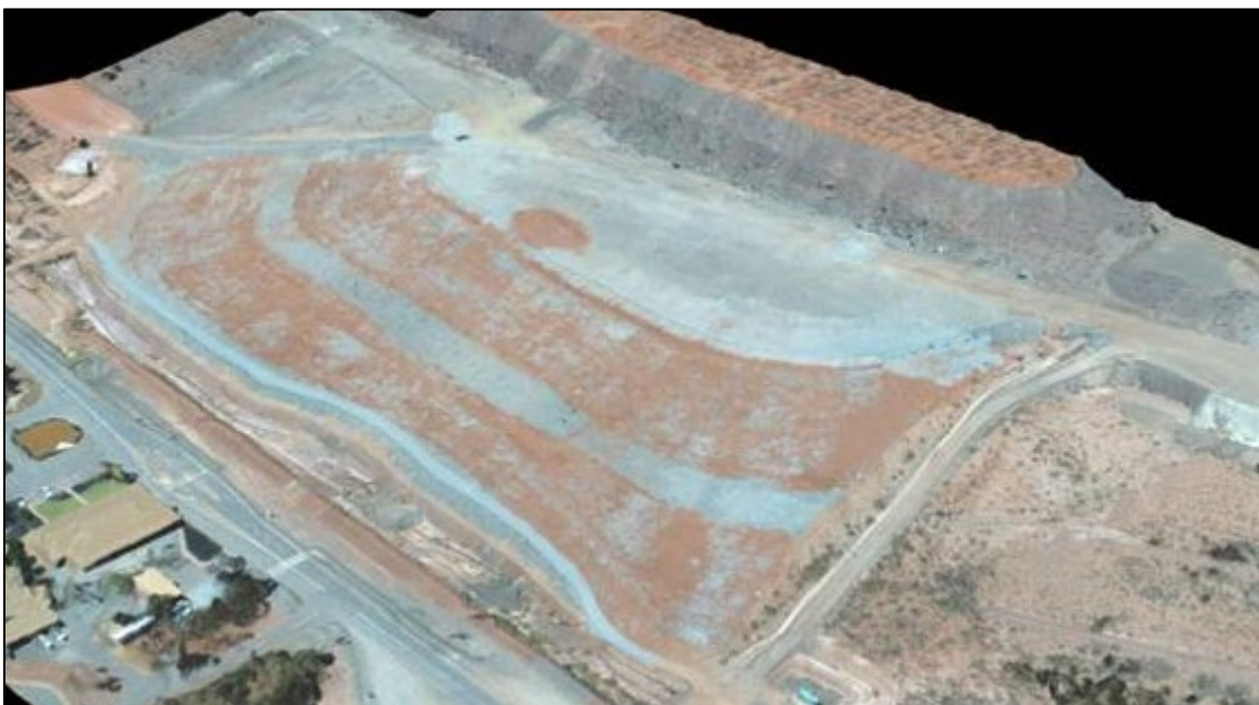
Figure 5-46: Old Croesus 2021 Capping and Completed Rehabilitation
