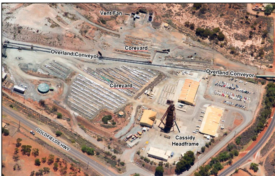
Figure 5-95: Mt Charlotte Surface Infrastructure
