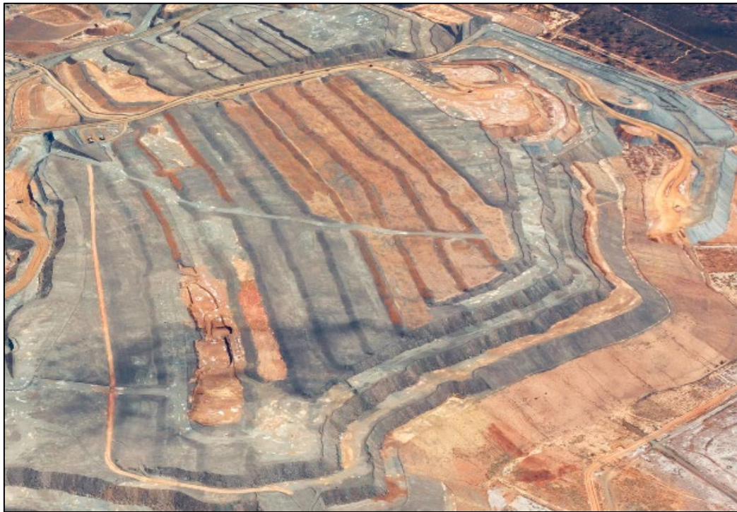
Figure 5-30: 5 m Lift Rehabilitation (2021)
