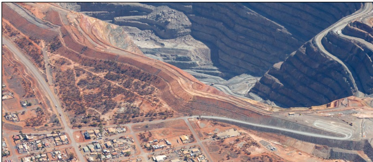
Figure 5-52: Southern Noise Bund (2021)
