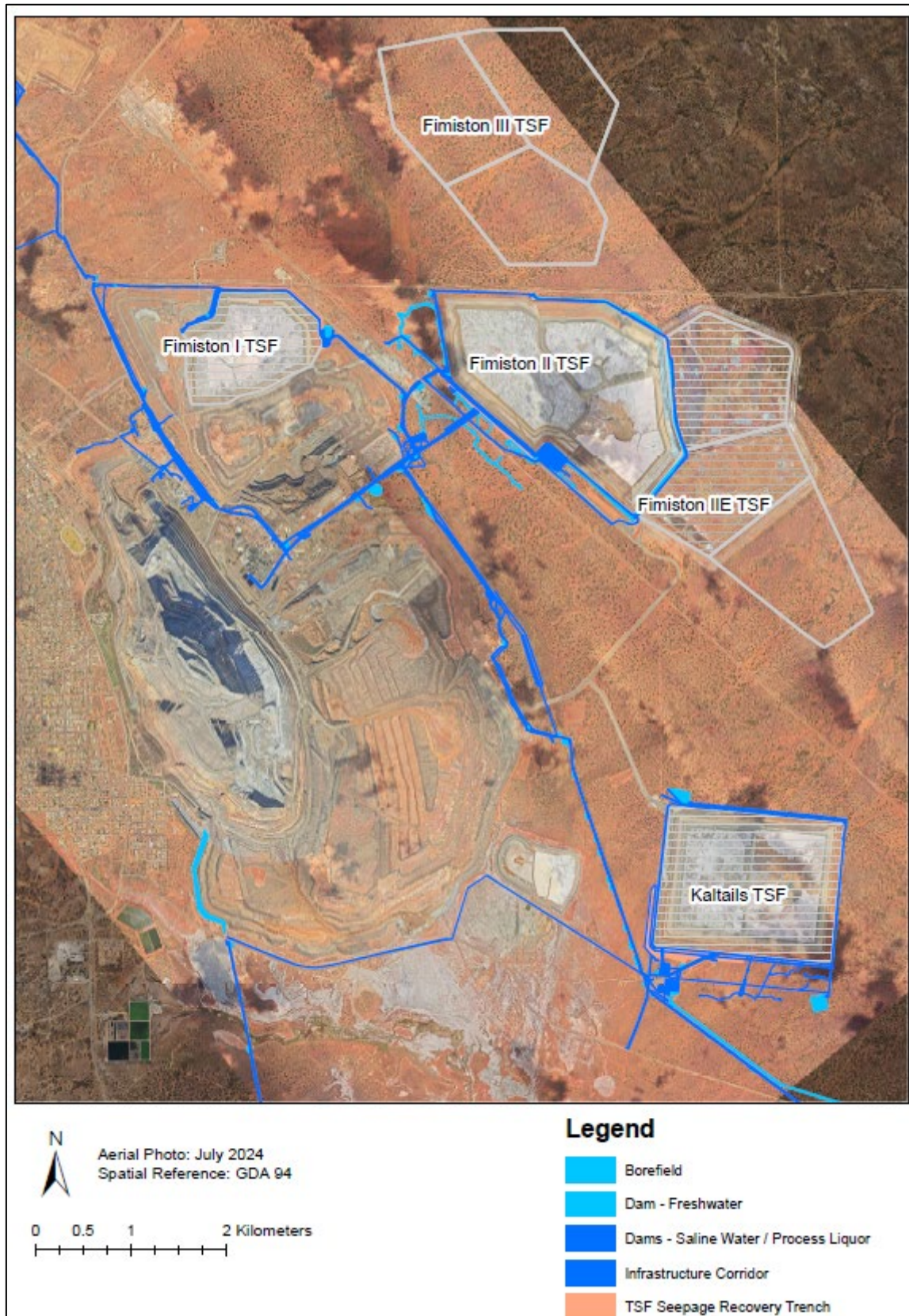
Figure 5-83: Water Containment Facilities Domain and Site Dams Feature
