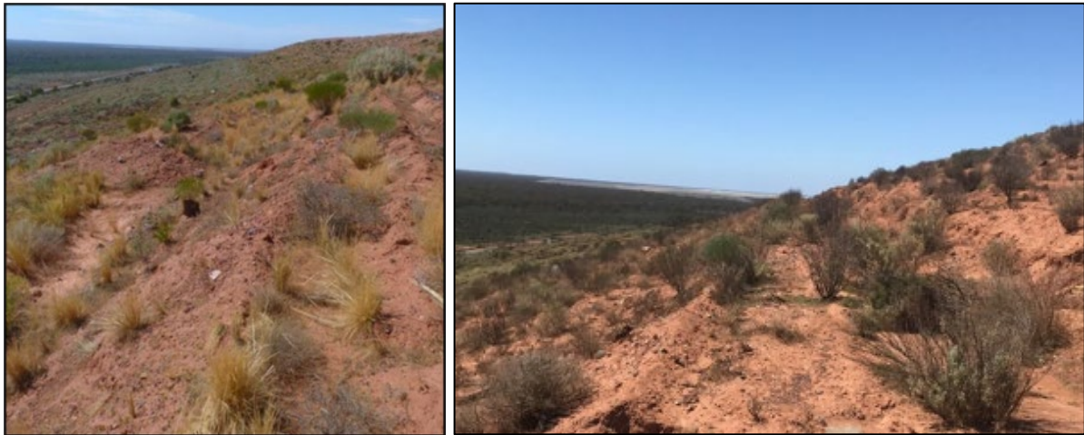
Figure 5-35: Oroya WRD Third Lift Eastern Batter – Status of Rehabilitation (2013 left and 2021 right)
