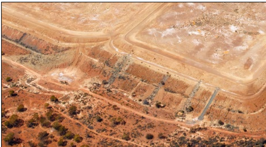
Figure 5-110: Erosion and Water Control Repairs on Mt Percy TSF Completed in 2019 (2021)
