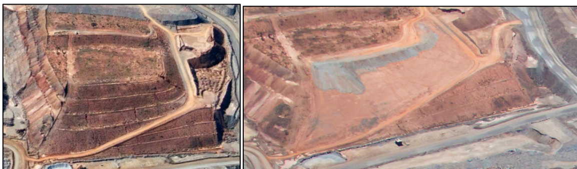
Figure 5-36: Radio Hill Prior to 2017 (Left) and during 2017 Remedial Works (Right)
