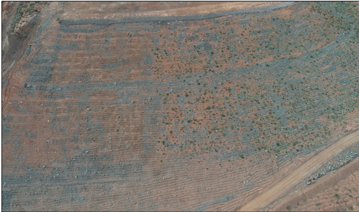
Figure 5-35: Radio Hill (2019) after remedial works (note vegetation difference between Class D (left) and Class A (right) soils)
