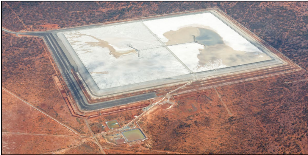
Figure 5-77: Kaltails with Buttress (2021)
