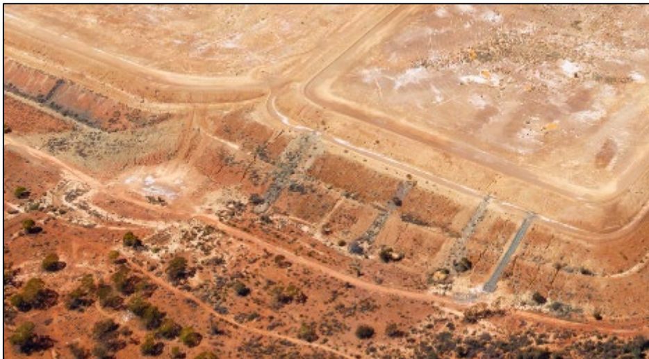
Figure 5-105: Erosion and Water Control Repairs on Mt Percy TSF Completed in 2019 (2021)
