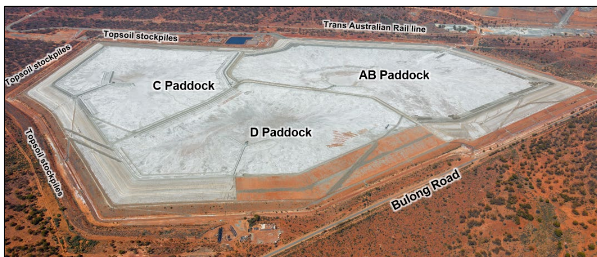
Figure 5-65: Fimiston II TSF, before buttressing (2021)
