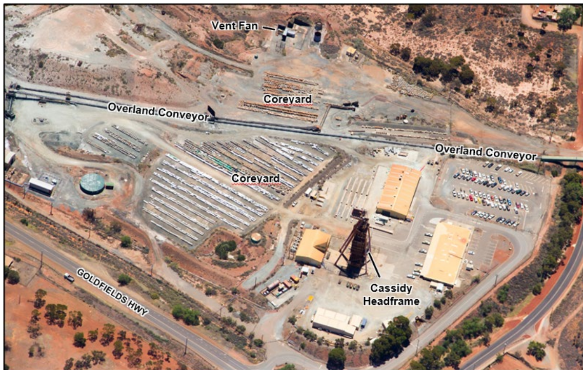
Figure 5-92: Mt Charlotte Surface Infrastructure
