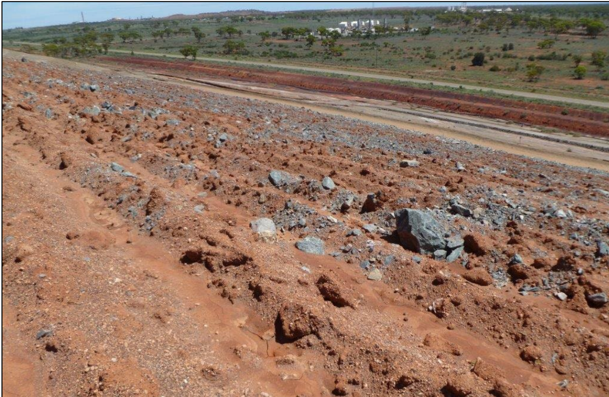
Figure 5-112: Fimiston I TSF Trial Immediately after Completion of Earthworks (Feb 2017)
