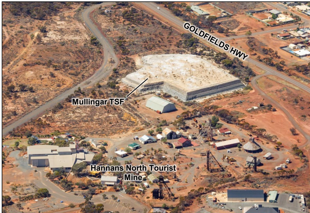
Figure 5-108: Mullingar Tailings Storage Facility (2021)
