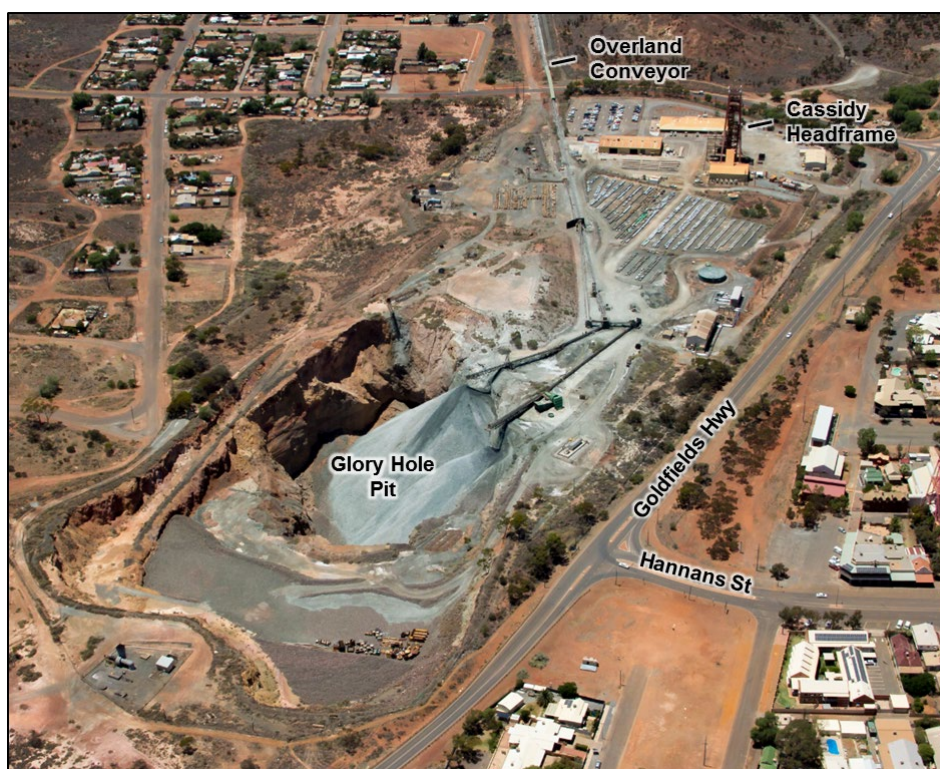
Figure 5-91: Mt Charlotte Mining Infrastructure
