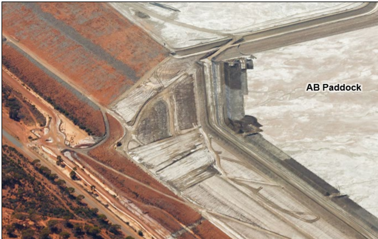
Figure 5-71: Fimiston II TSF 2021 commencement of reshaping of AB Paddock
