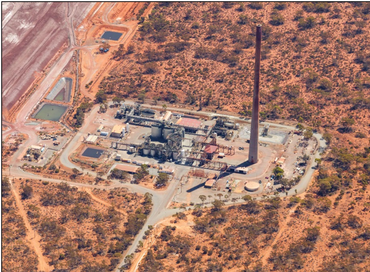
Figure 5-83: Gidji Processing Plant (2021)
