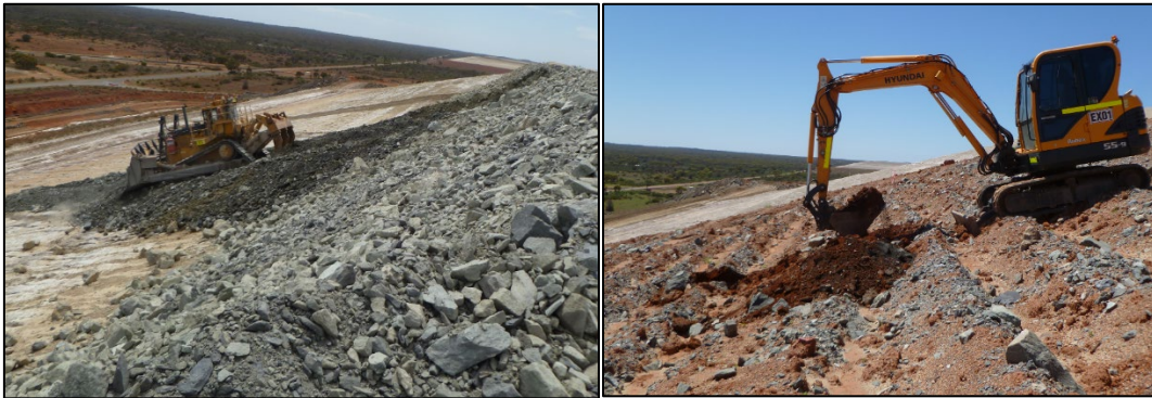
Figure 5-61: Fimiston I TSF Trial Earthworks in Progress (2016 and 2017)
