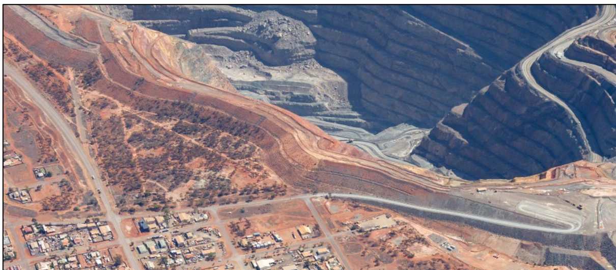
Figure 5-50: Southern Noise Bund (2021)
