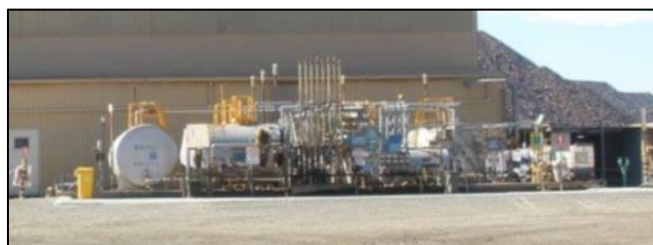
Figure 5-22: Fimiston Mining Maintenance Workshops Main Hydrocarbon Area
