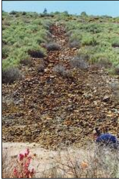
Plate 10: Black Flag Beds in Dump Drainage Structure, Mount Percy
