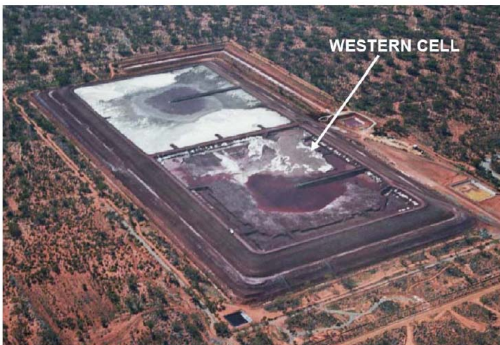
Figure 1.8. Gidji Tailings Storage Facility
