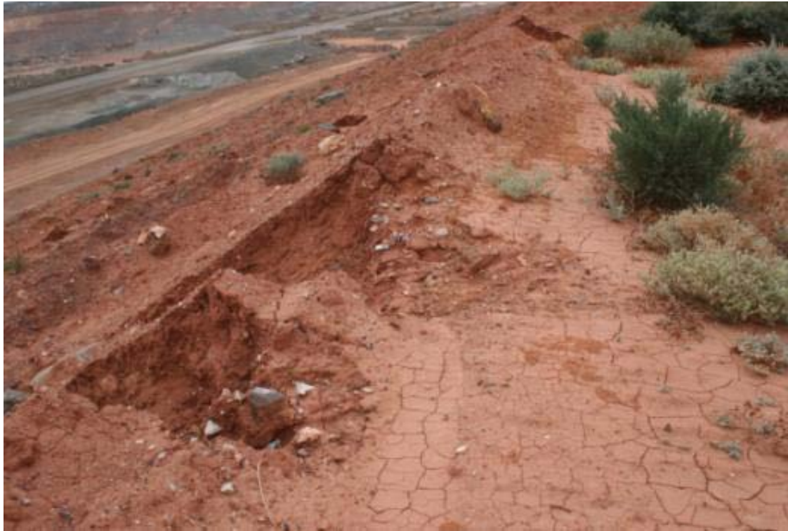
Figure 24: Break in Berm on Second Lift (Near Radio Hill Transect 3)
