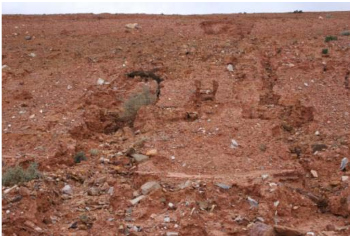
Figure 25: Tunnelling down slope from break in berm near Transect 3
