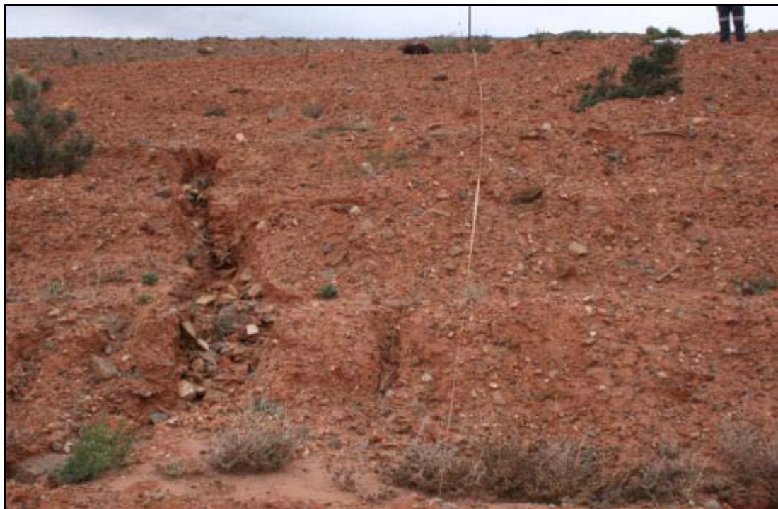
Figure 9: OTD Area Transect 1 View from Bottom 2009.
