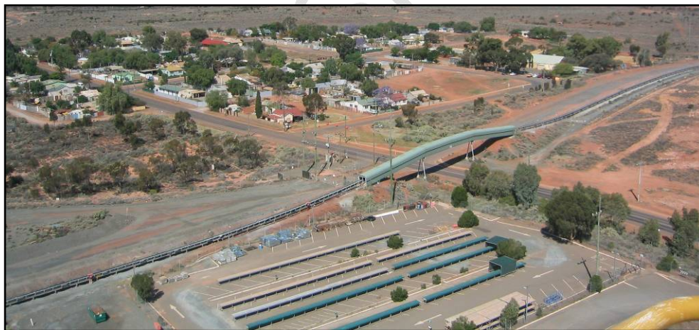
Figure 4 Fimiston to Mt Charlotte Overland Conveyor
